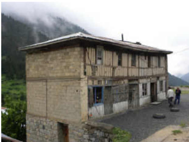
Teehaus in Sivri Kaya
